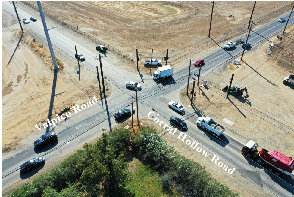
IMAGE: Construction Site
